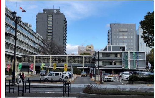
Hiroshima Prefectural Office
